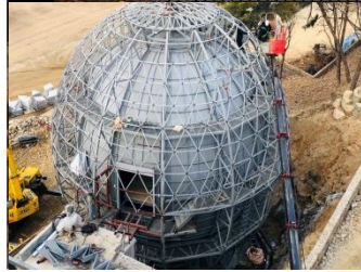
360 Dome installation ( triangle frame )
