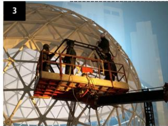
Projection bracket installation
