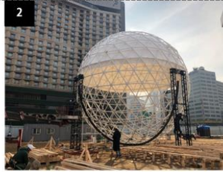
Dome construction ( frame )
